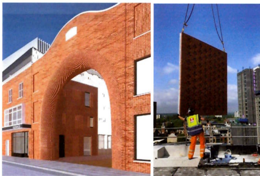
Figure 18 –Moore Street Archway & Typical Precast Panel Installation
