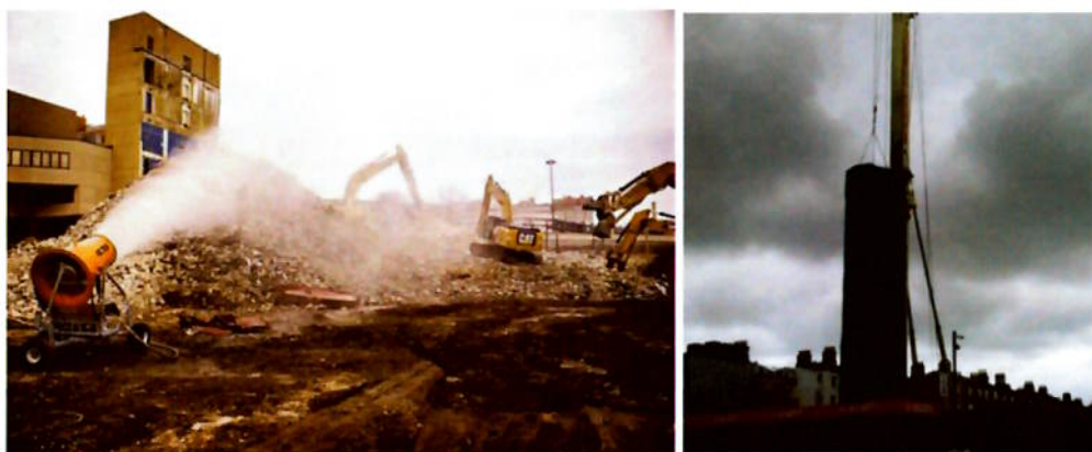
Figure 40 – Typical Dust Mitigation Measures
