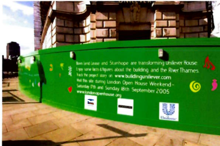
Figure 5 Typical Pavement Hoarding with Street Lighting
