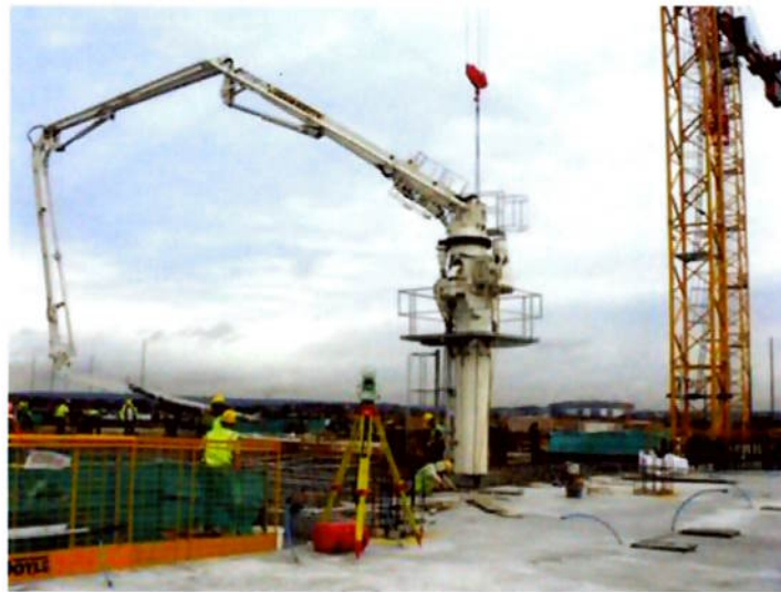
Figure 15 - Typical Concrete Placement
