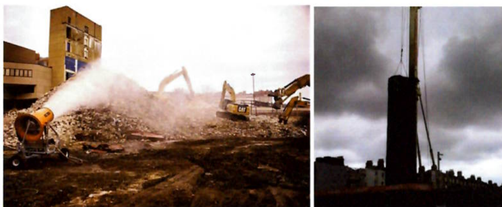
Figure 27 – Typical Dust Mitigation Measures
