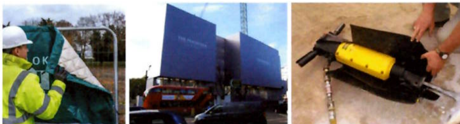
Figure 39 – Typical Noise Mitigation Measures
