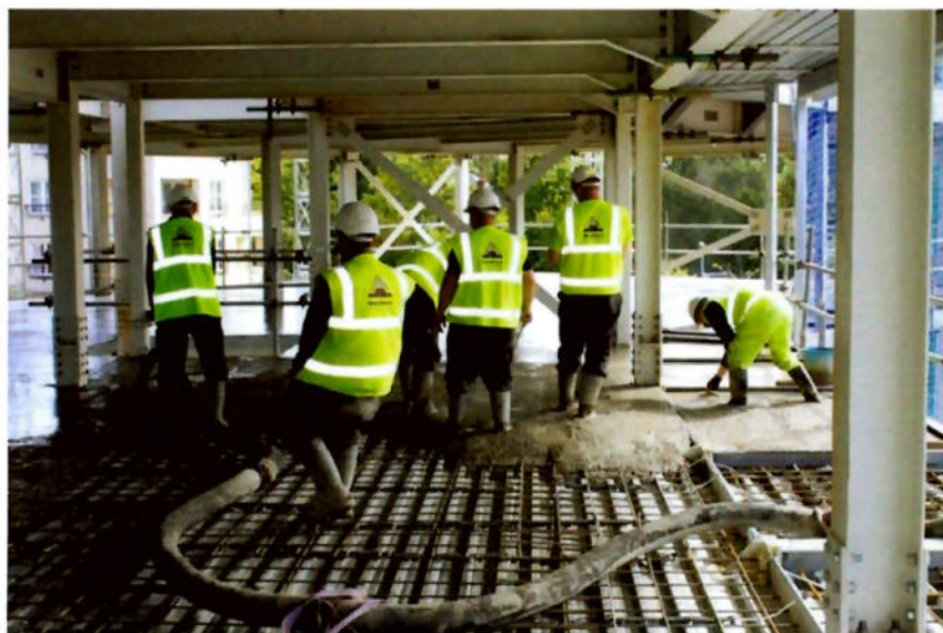
Figure 17 – Typical Concrete Pour on Metal Decking
